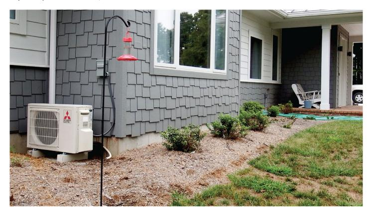
Managing humidity is difficult but the way the ductless mini-splits run helps with humidity by running at a lower speed with fewer stops and starts – which also helps with the equipment's long-term durability."
