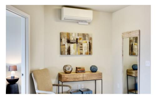
selection was about performance and control. There's really not any other way to deliver cooling close to this cost other than packaged terminal heat pumps, but those don't deliver on performance. And we'd worked with ductless heat pumps before, so we knew the technology works."
